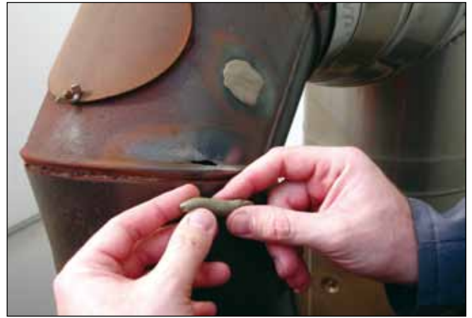
Repair of an outgoing air pipe
