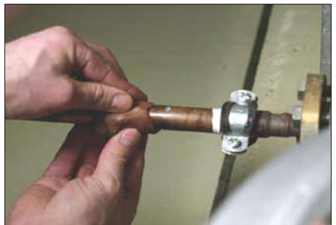
Sealing of a copper tube
